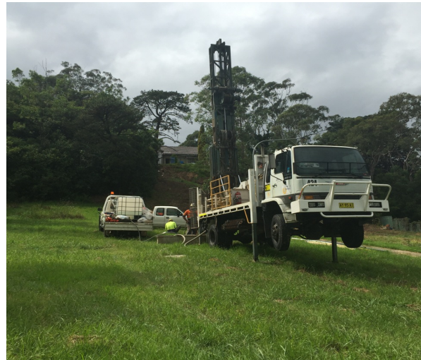
Plate 4 – (13/3/15) Drilling rig at BH9
