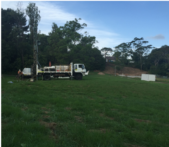
Plate 3 – (12/3/15) Drilling rig at BH8
