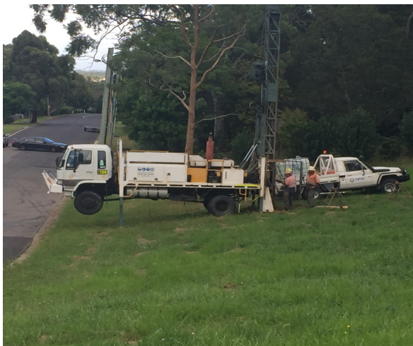
Plate 5 – (14/3/15) Drilling rig at BH11
